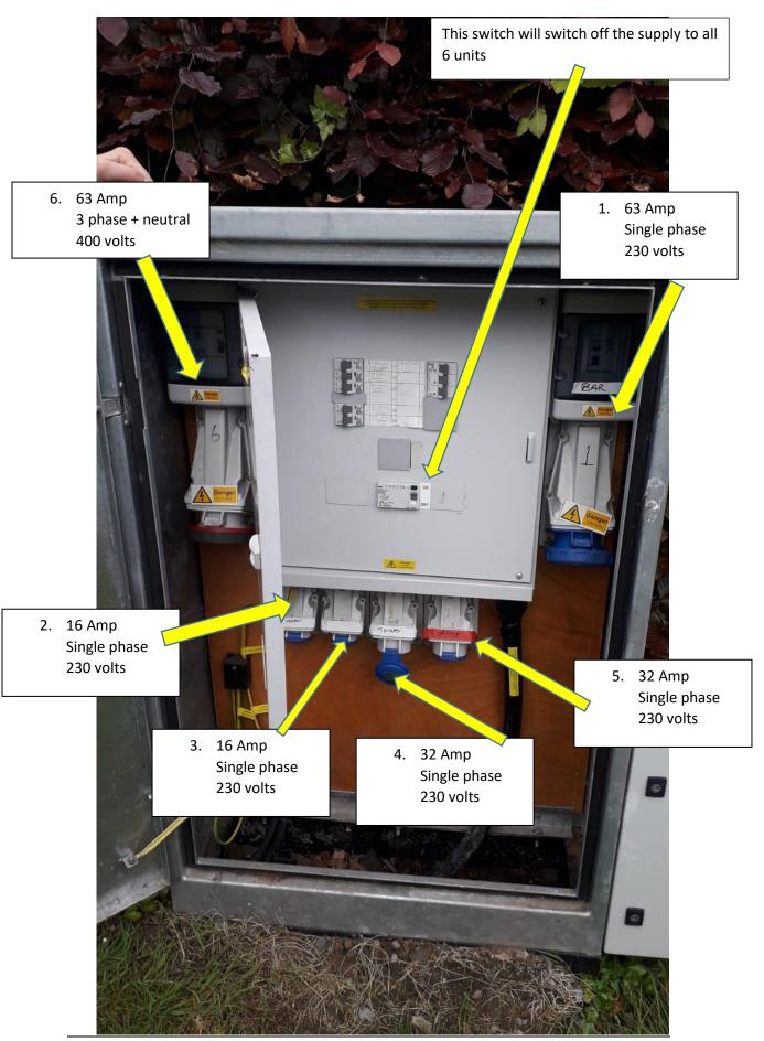
Safety hatch at the bottom is to allow the box to be **locked** during use for health and safety reasons.
