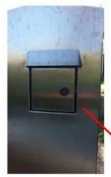
The housing for the manual over-ride switch is located on the <u>side</u> of the cabinet at the far right-hand end of the bridge as shown below.
