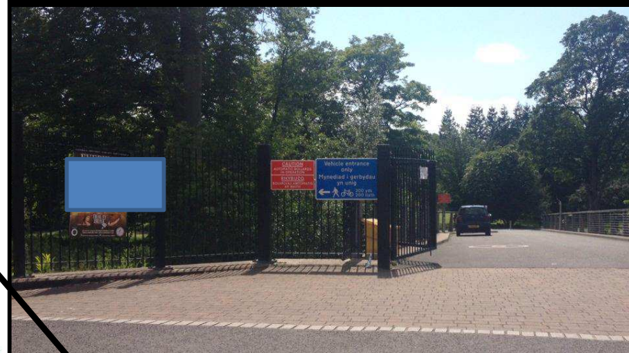
4. Vehicle Access Bridge – On North Road
