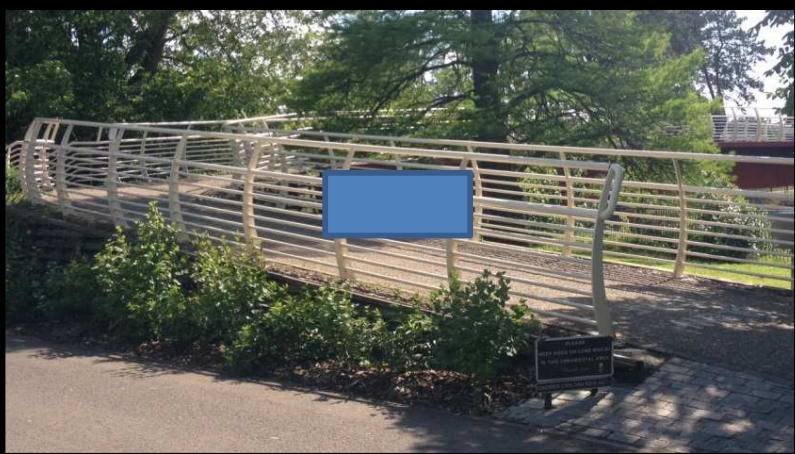
3. Millennium Bridge – Opposite Summerhouse Cafe
